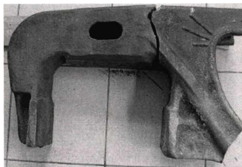
Fig. 1. Fracture of the side frame in the area of the axle box opening
